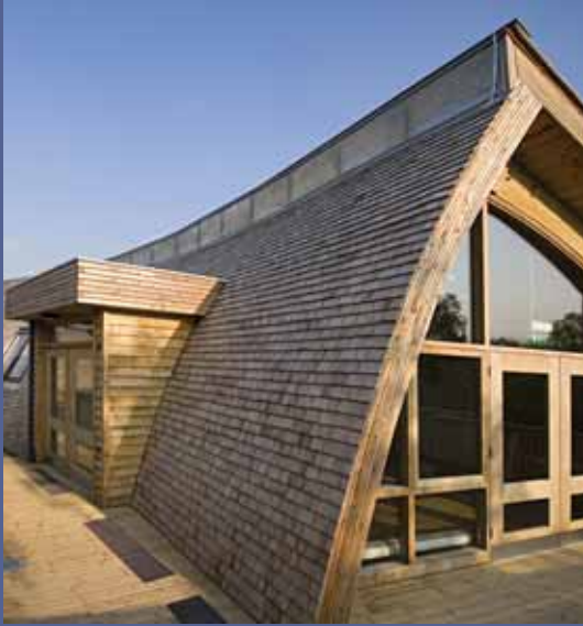
High-quality, sustainable design at Shorne Woods Country Park visitor centre, Gravesend
