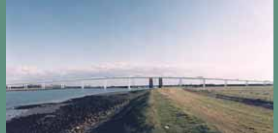
The new Sheppey Crossing improves access between Sheppey Island and Kent
